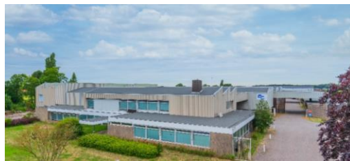
Plasthill Warehouse & Distribution
